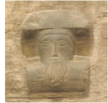
Figure in middle of Clerestory Wall
